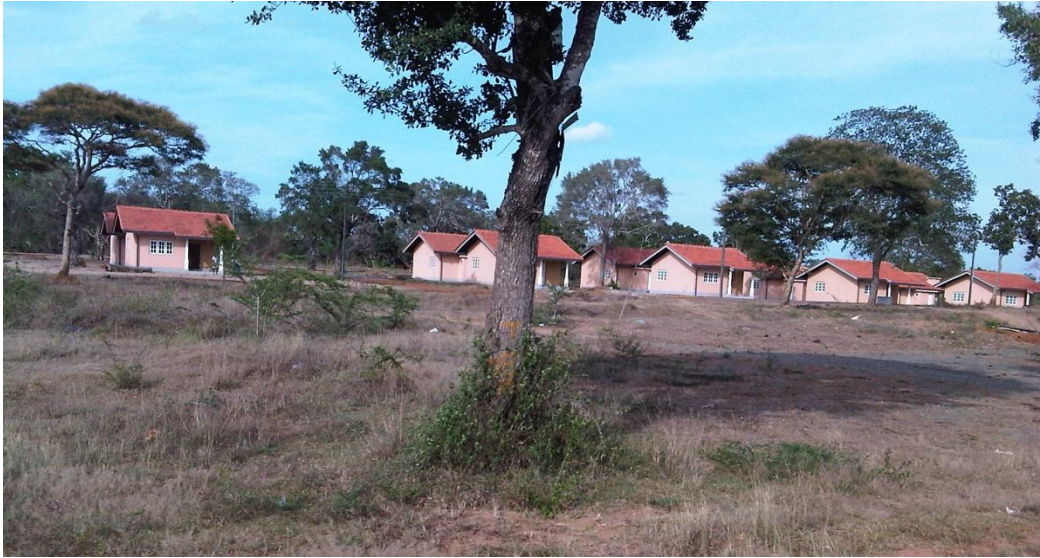
Houses built along the Madhu Road by Bank of Ceylon, 50 houses of which 45 are allocated to Sinhala families and 5 to Tamil families
